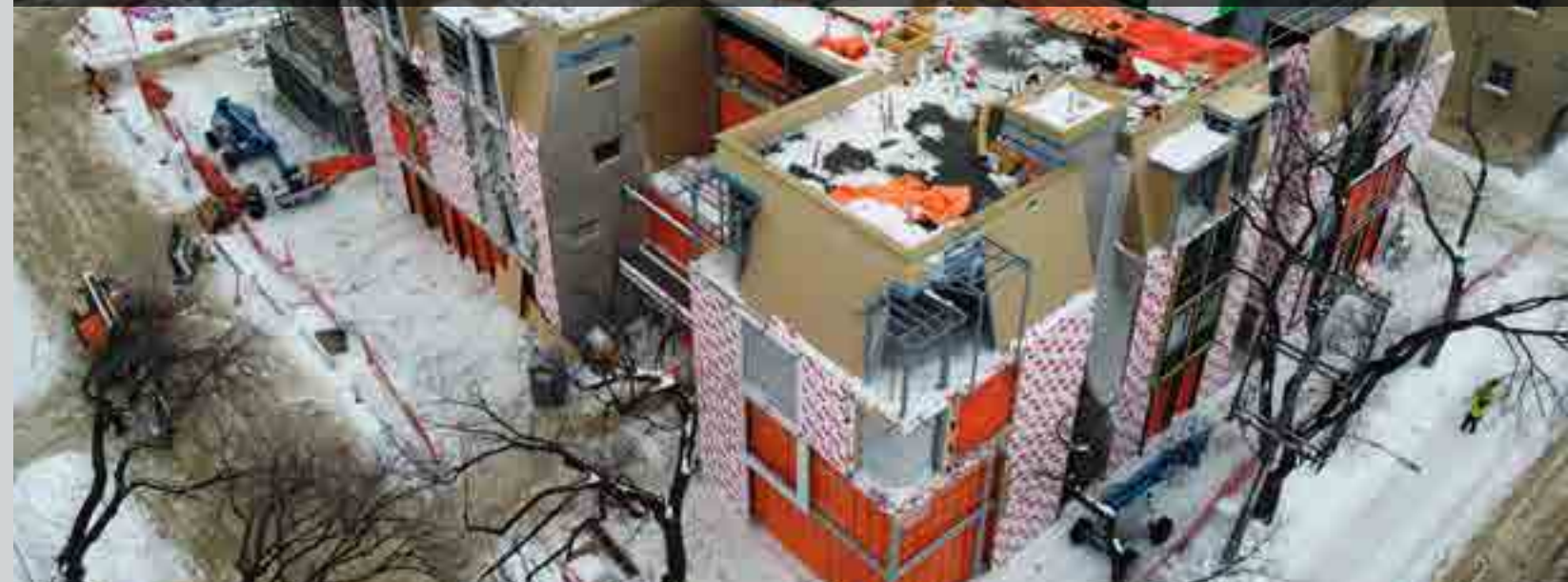
The new Ronald McDonald House construction site at 62 Juno Street
